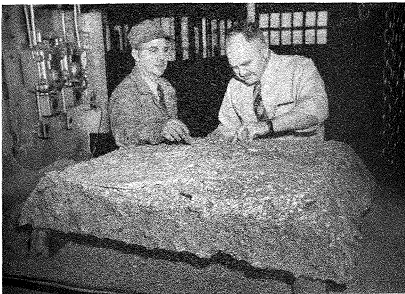
Senior tester Roscoe Rush and Harold Garman inspect a ferro-chrome cast after it has had one pass in the Wheelabrator abrasive blast. This one-ton cast was sent in by the Vanadium Co. of America, Niagara Falls, N. Y., to determine the effectiveness of the Wheelabrator to remove the scale.
